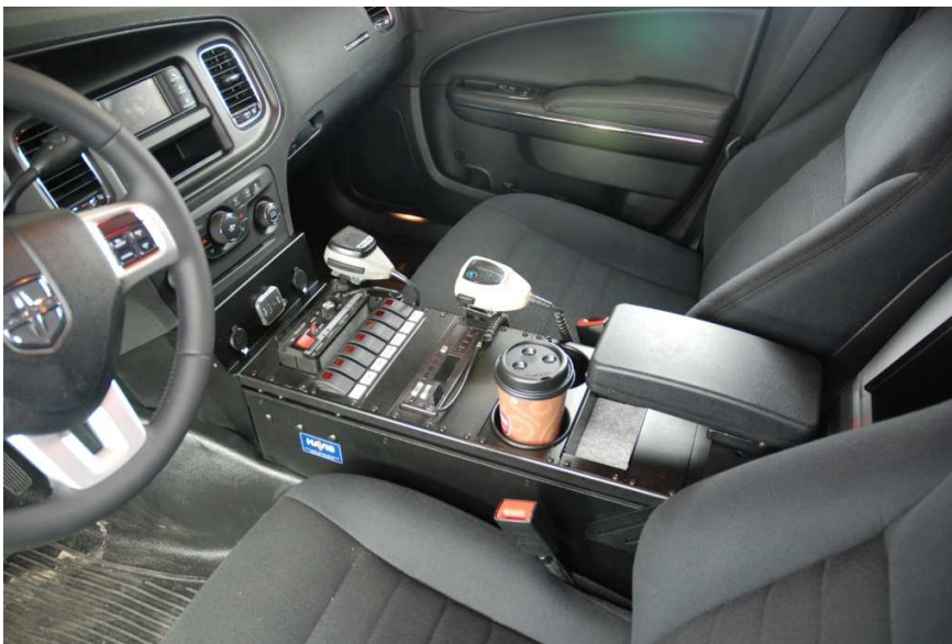
Completed console installation (example 3)
