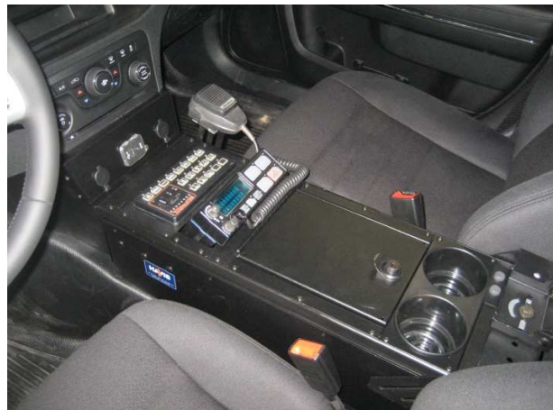
Completed console installation with Self Contained Radio and accessories. (example 2)
