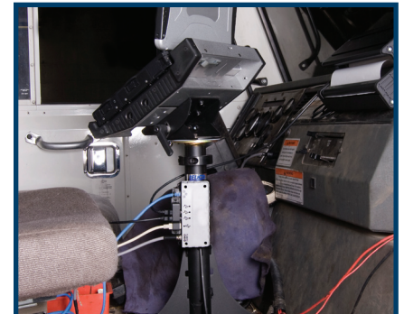
Rugged Communications Hub mounted inside a municipal services vehicle
