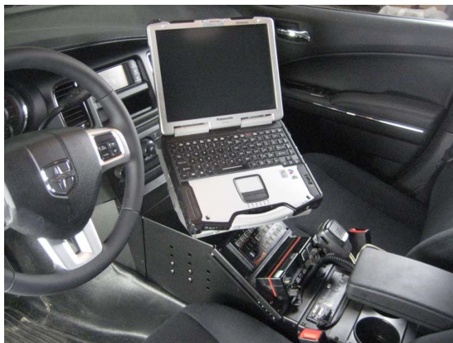
Completed C-VS-0809-CHGR-1 console installation with Laptop / Docking Station (example 2)
