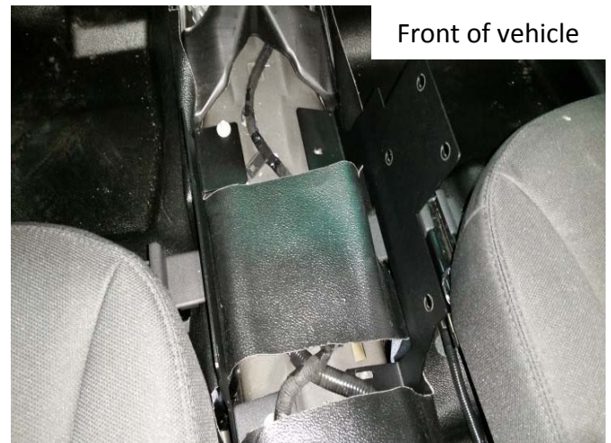
Bolt driver and passenger side front hump brackets to floor with previously removed OEM floor bolts.
