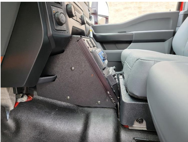
Wire, mount and install equipment prior to reinstalling OEM center seat.
