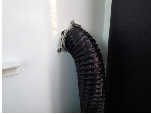
Attach supplied vent hose to vent adaptor and round vent with supplied hose clamp. Hose needs to be cut into two (2) 3 foot pieces.
