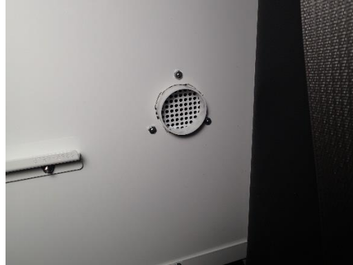
View of vent adaptor from front side.
