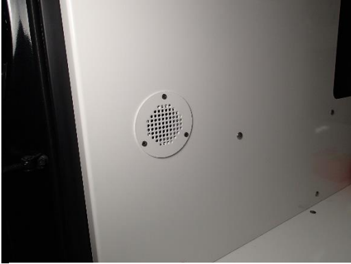
Attach round vent adaptor to front wall using three (3) #10 x 1/2" flat head screws and keps nuts.
