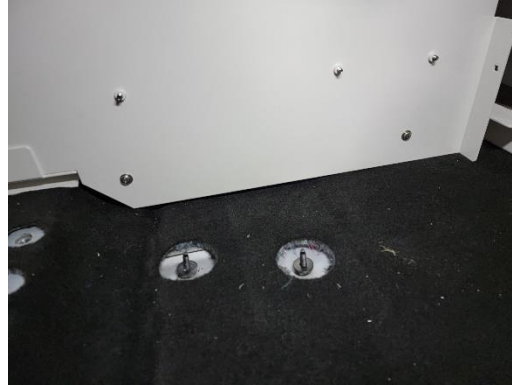
Attach to floor using 1/4" x 3/4" Phillips head bolts and flat washers.
