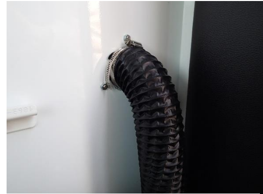
Attach supplied vent hose to vent adaptors with supplied hose clamps. Hose needs to be cut into two (2) 3 foot pieces.
