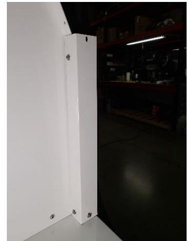
Loosely attach K9 lower side filler panel to rear wall with 1/4 x 3/4 Phillips pan head bolts and washers.
