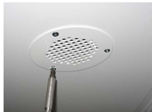
Align the three mount holes of the vent adapter cover with the pre-punched holes in ceiling. Attach each vent to ceiling using #8 x 3/8" flat head sheet metal screws. (Screws included with standard insert hardware)
