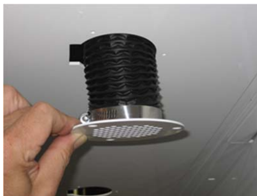
Route hose into ceiling holes and cut off any extra slack.. Attach the hose to the vent bracket using a 3" hose clamp
