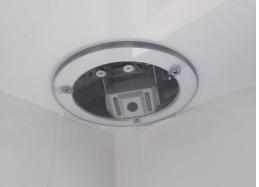
Mark holes on the ceiling and predrill with 1/8" drill bit. Reposition camera assembly and mount using #10 x 3/4" Flat head sheet metal screws.
