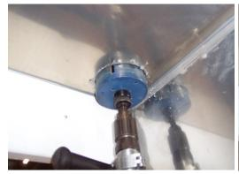
Determine mounting location for camera and mark hole. Be sure to make sure the polycarbonate dome cover fits properly before drilling 4 ½" hole. Take caution not to drill into any wires.
