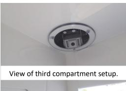
Note: Cameras come standard with night vision LED lighting. However the night vision LED does not work correctly because of reflection off of the ceiling mounted vandal proof guard.
