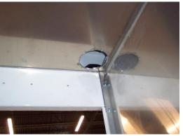
Once hole is drilled, deburr the metal. Reach through the opening and pull the camera cable through the opening.
