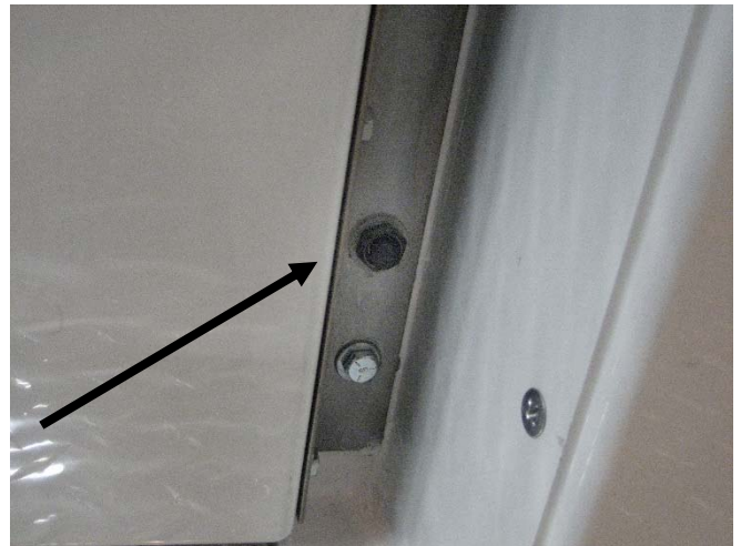
Mark the door frame roughly 2" above the lowest door hinge bolt
