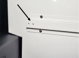
Attach side-mounting brace to the horizontal back support of the K9-F28 insert using 1/4" x 3/4" bolts and washers.
