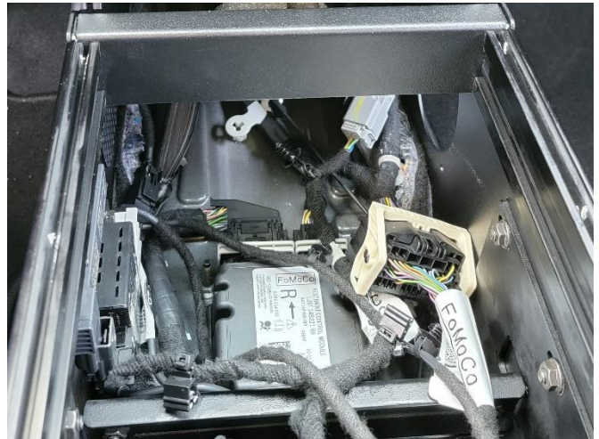
Reinstall previously removed interior OEM console items.
