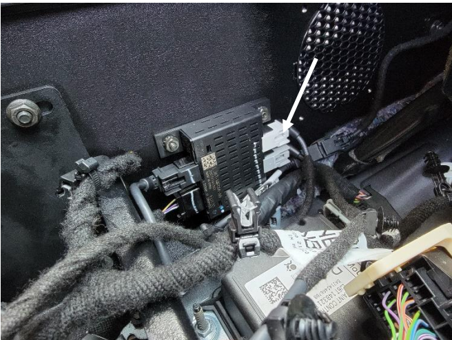
Plug modules back in that had been relocated to side the of the console.
