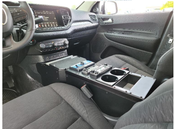
Wire and install all equipment.
