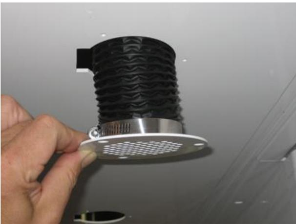
During transport insert installation you will be prompted to return to the PT-A-501 instruction to attach the hose to the vent adapter brackets. Route hose into ceiling holes and cut off any extra slack.
