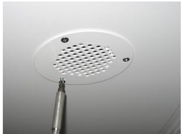
Align the three mount holes of the vent adapter cover with the pre-punched holes in ceiling. Attach each vent to ceiling using #8 x 3/8" flat head sheet metal screws.
