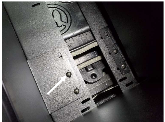
Attach rear of console housing to floor bracket with 1/4" x 3/4" carriage bolts and serrated nuts.
