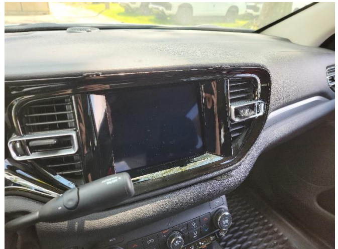
Reinstall previously removed dash trim and instrument cluster.
